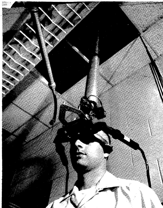
FIGURE 4—The ultrasonic head position sensor in use
